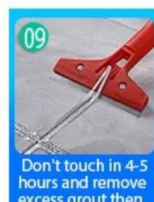
Don't touch in 4-5 hours and remove excess grout then.
